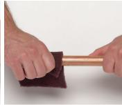
Following tube preparation steps 4 to 8 in the RLS installation instructions is important for preventing leaks.
