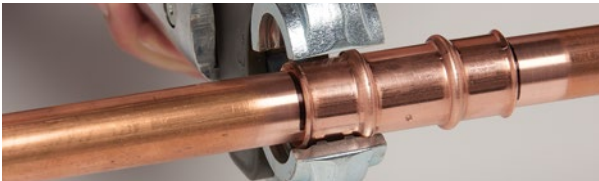
1. Insert the tube in the fitting
