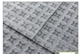
Roll joints without cross joints
