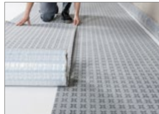
Roll with 1.9 in (5 cm) minimum overlap on longitudinal edge
