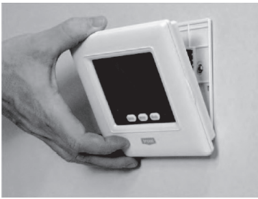
Fig. 4 - Attach Thermostat to Backplate
